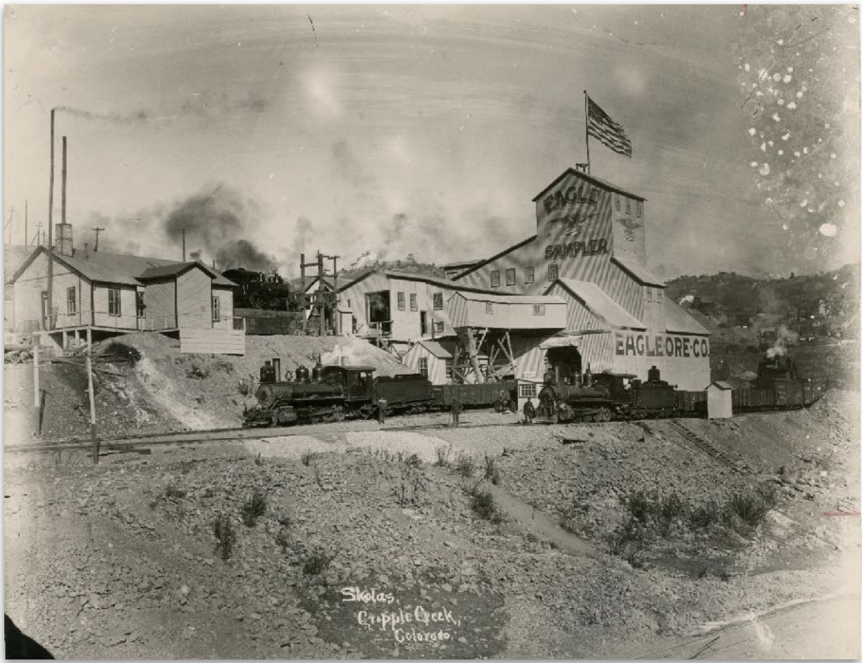
Figure 3. The Eagle Company Ore Sampler near Victor, Colorado, which served the regional mines by doing assays of the ore from mines to determine worth and content. The sampler also bought ore. Undated photo by Julia Skolas. Courtesy of the Cripple Creek District Museum. CCDM 009.
