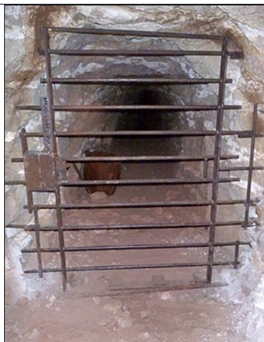
ABOVE: Bat gate installed during 2009. Photo courtesy of National Park Service Resource Management.
