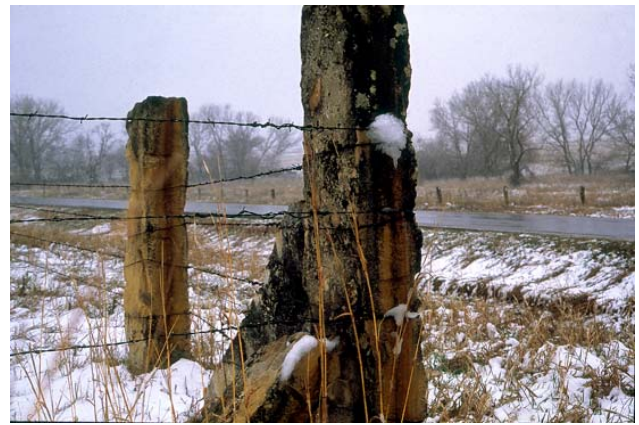
Fig. 3. Stone fence posts quarried from the "fencepost limestone member" of the Greenhorn Limestone. Early settlers in Kansas noted a shortage of trees suitable for fence posts so used available material--stone. Photo courtesy of Kansas Geological Survey.
